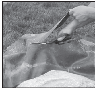
Trim off any excess liner.
