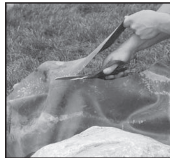
Trim off any excess liner.
