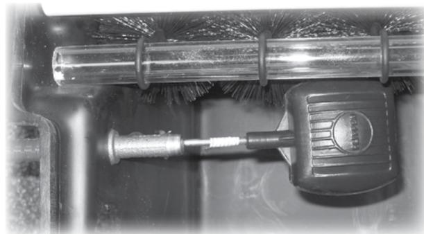
**WFS37** — Install the autofill in the back wall of the skimmer by drilling a  $\frac{3}{4}$ " hole 3" down from the top of the skimmer. The auto fill is usually located in the back wall of the
