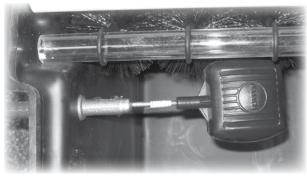
WFS37 — Install the autofill in the back wall of the skimmer by drilling a <sup>3</sup>/<sub>4</sub>" hole 3" down from the top of the skimmer. The auto fill is usually located in the back wall of the
